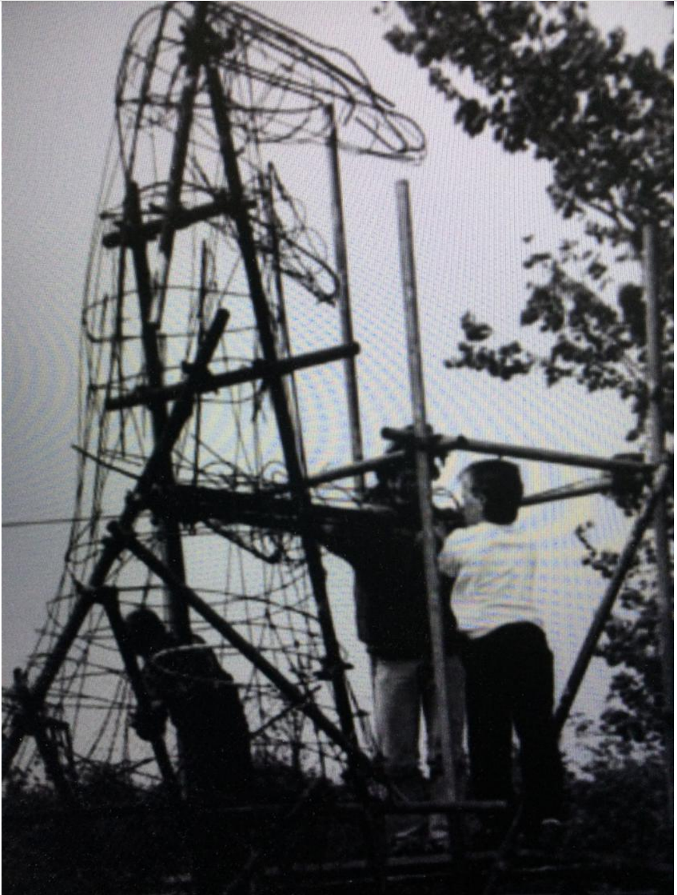
7. Image 2 Scaffold pole and wire construction. / 21 Mar 2022
