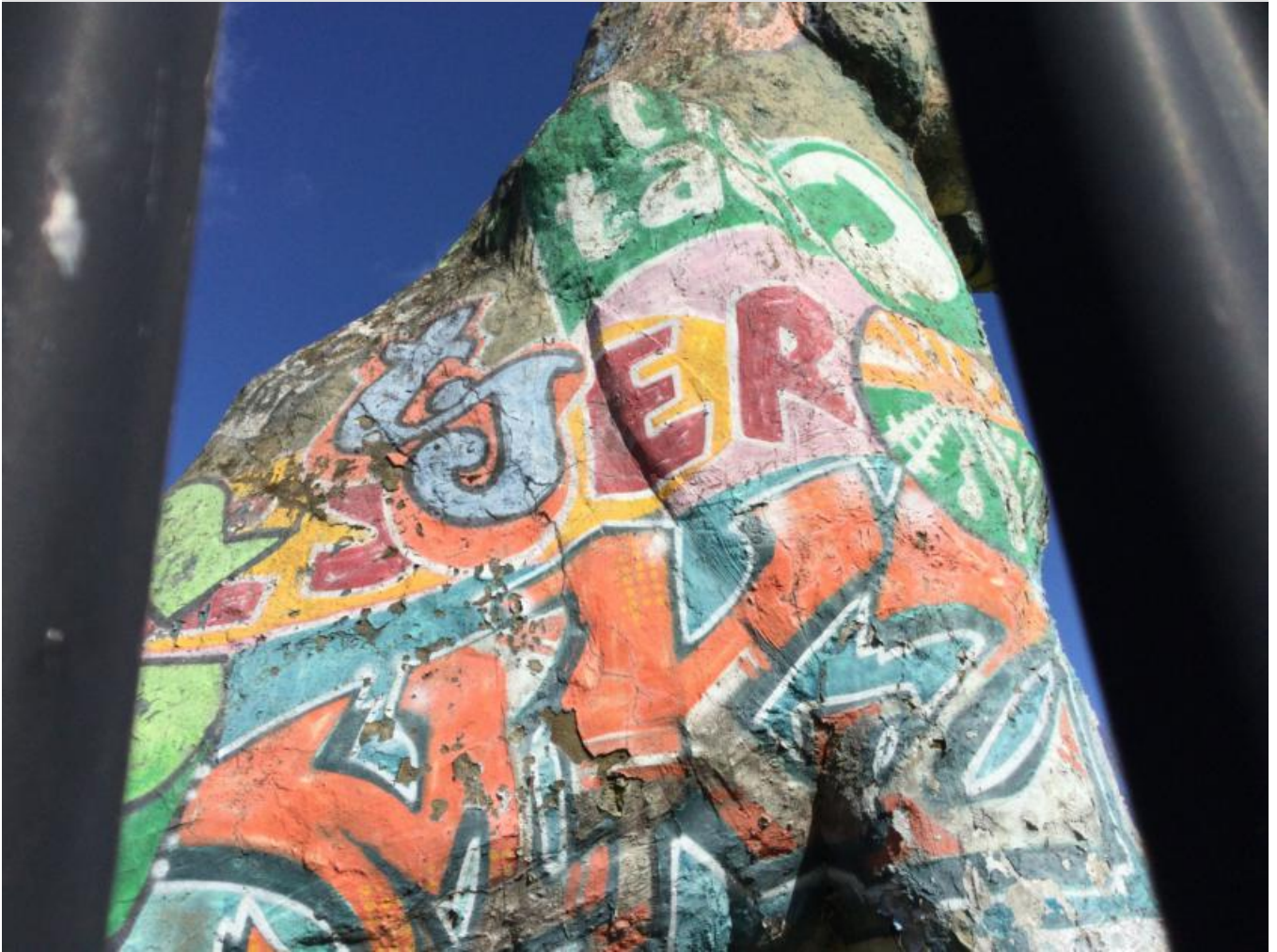
13. Image 14 Fissures Graffiti / 21 Mar 2022
