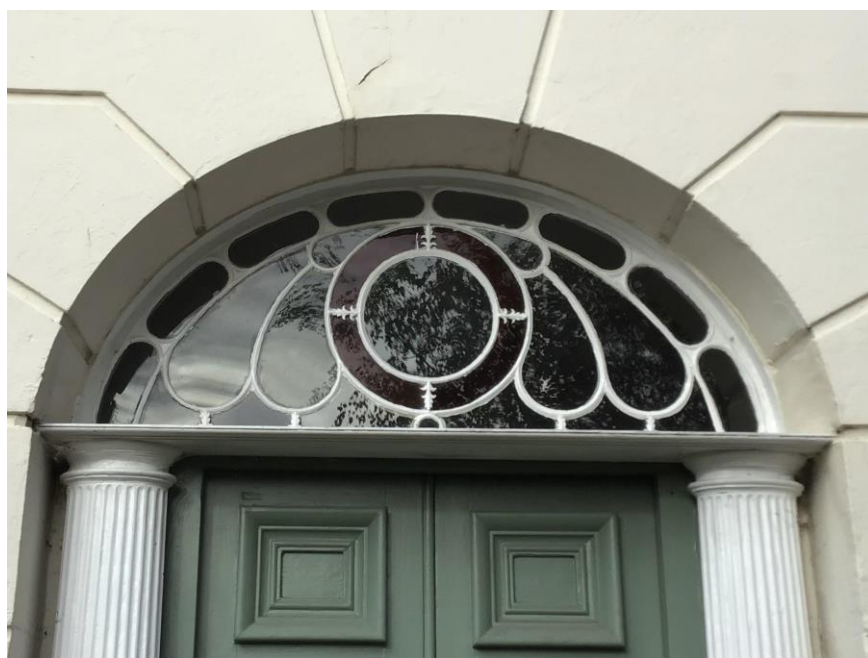
Simpson House: front door with fanlight
