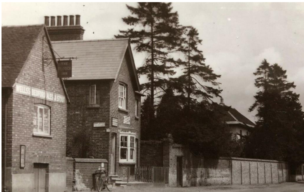
A view along Simpson Road showing the high brick wall which formerly enclosed the gardens
